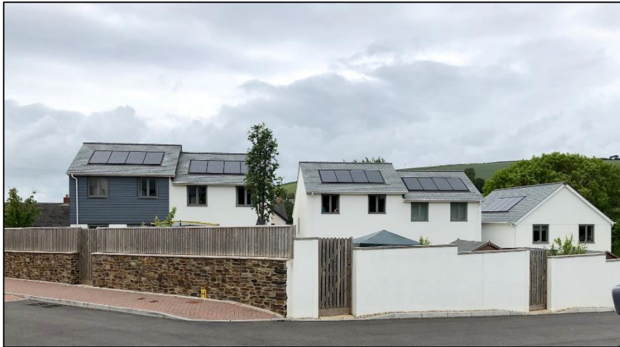
Photovoltaic panels at Creek Close, Frogmore
